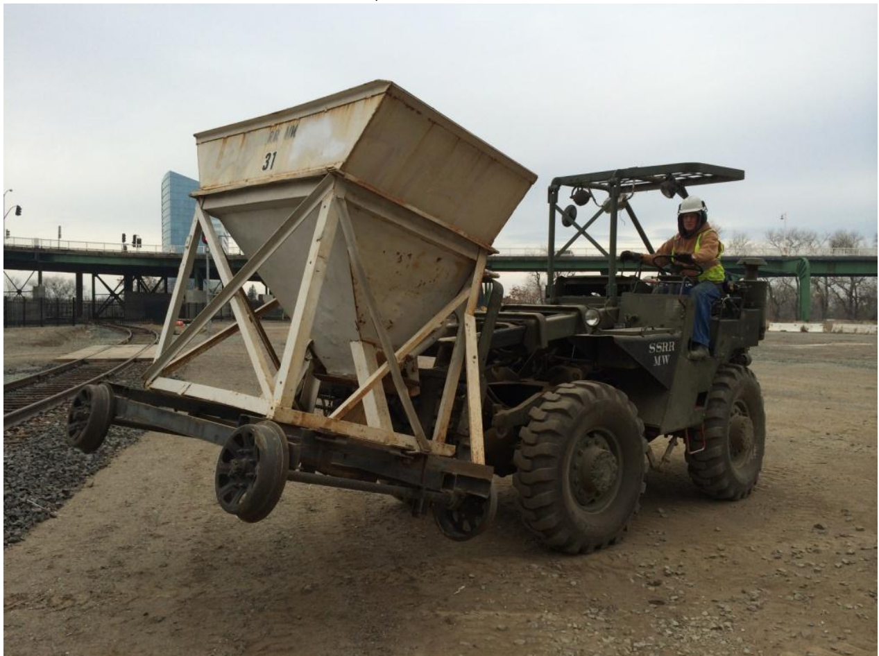
Steve on Big Green moves a ballast hopper onto the track
