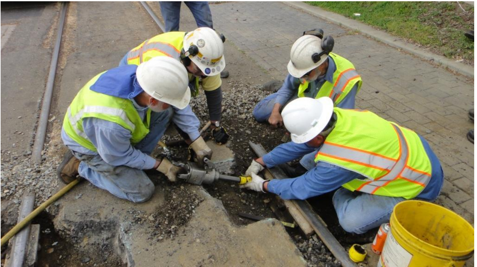
Mike M., Mike F., Alan, and Scott make a second attempt with the impact wrench to free the nut from the bolt.
