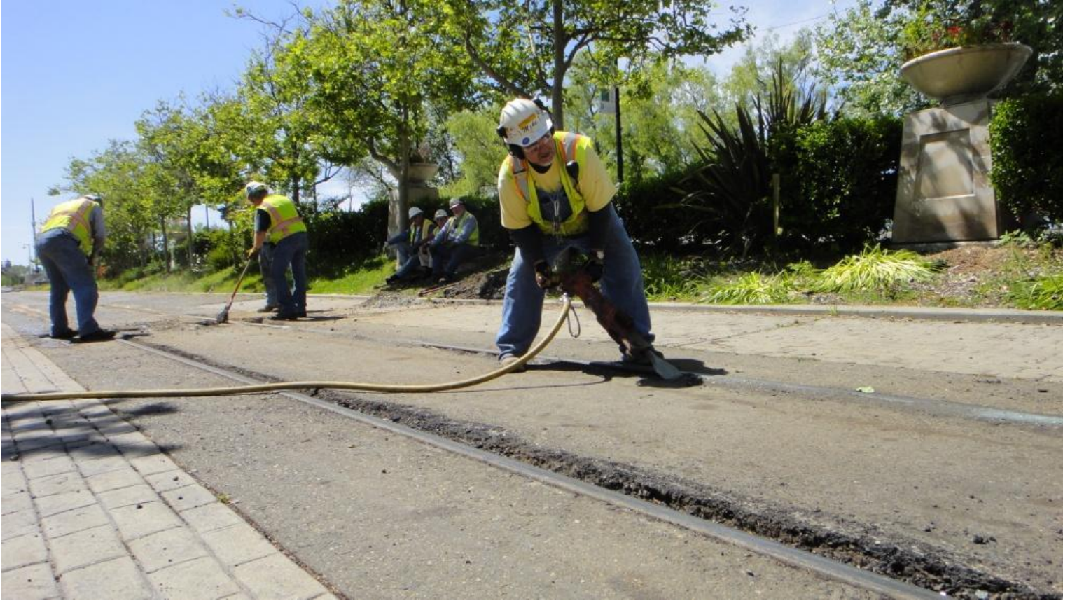
Mike F. uses the jackhammer to shave the buckling asphalt
