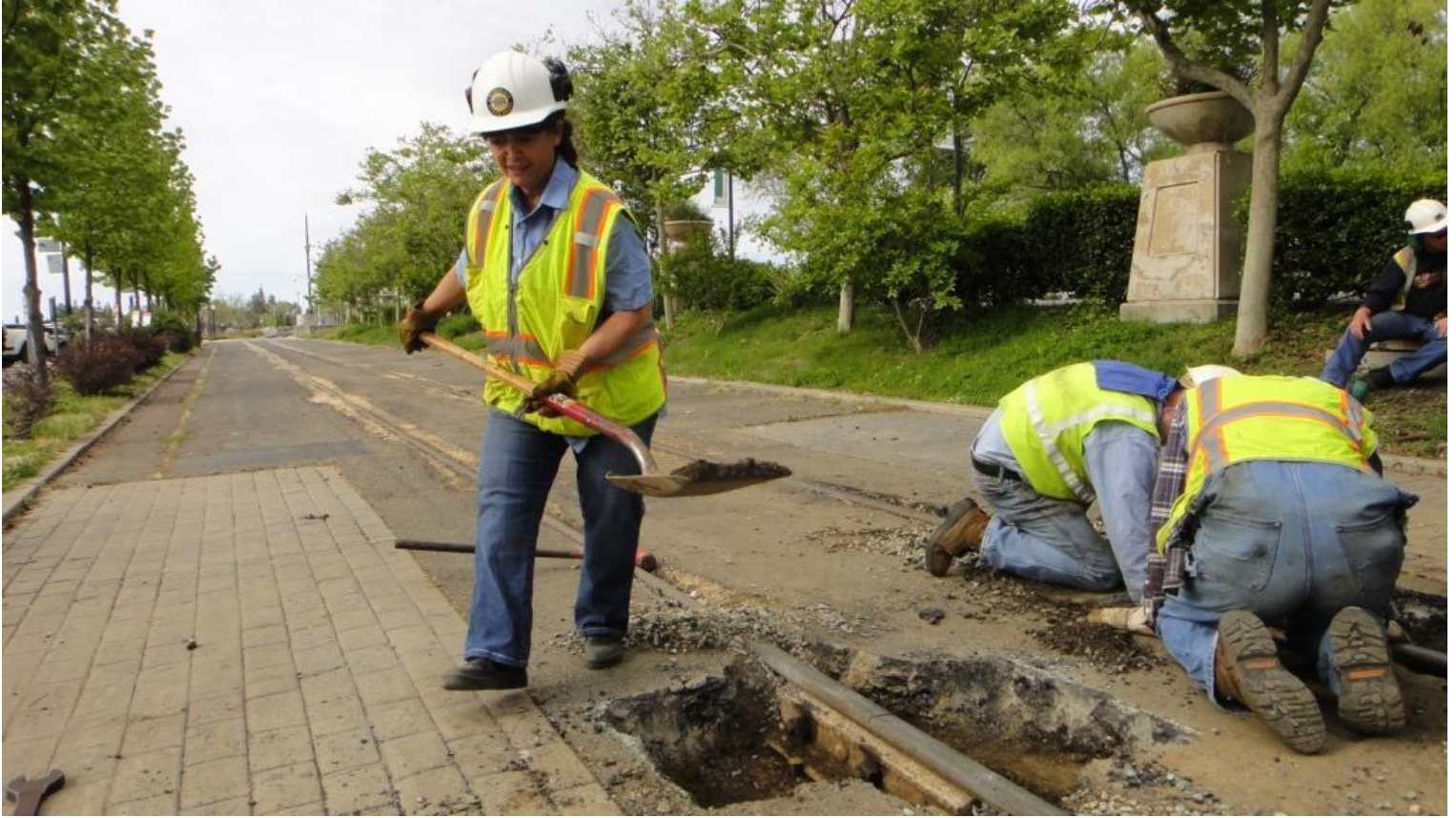
Meanwhile, Pam continues digging out the joint opposite
