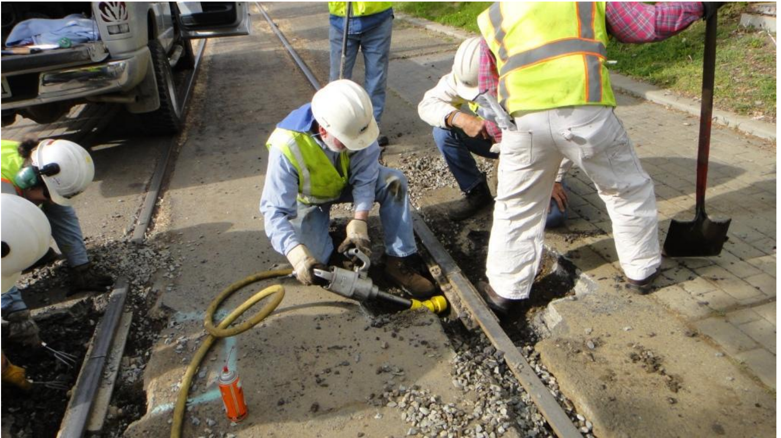
The impact wrench is brought in. Mike M. tries to get a grip on the nut while Mike H. holds the bolt in place with his foot
