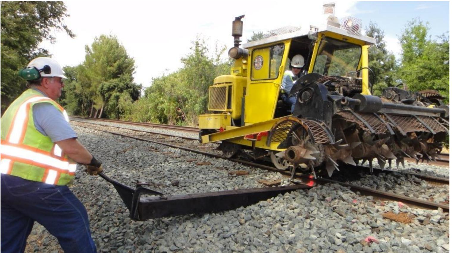
One final duty. Chris guides a new tie into position while Heather manages the scarifier-inserter
