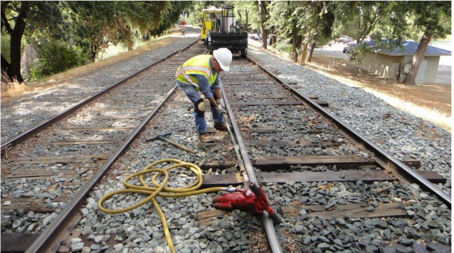
Mike T. uses a lining bar to straighten a wayward spike
