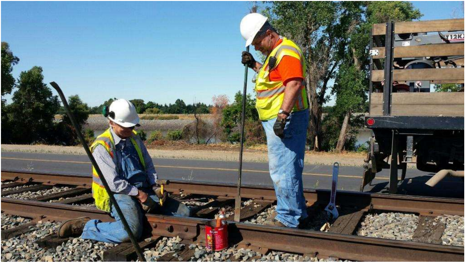
Steve and Mike F. replace lock-washers on several joints
