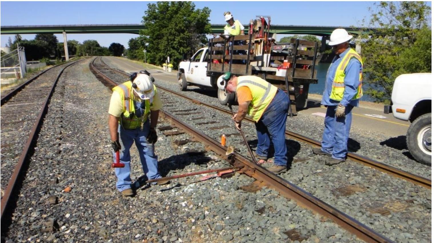
At Mile Post 1.1, Frank loosens the bolts in the joint so that Mike F. could use a lining bar to line-up the bolt-holes
