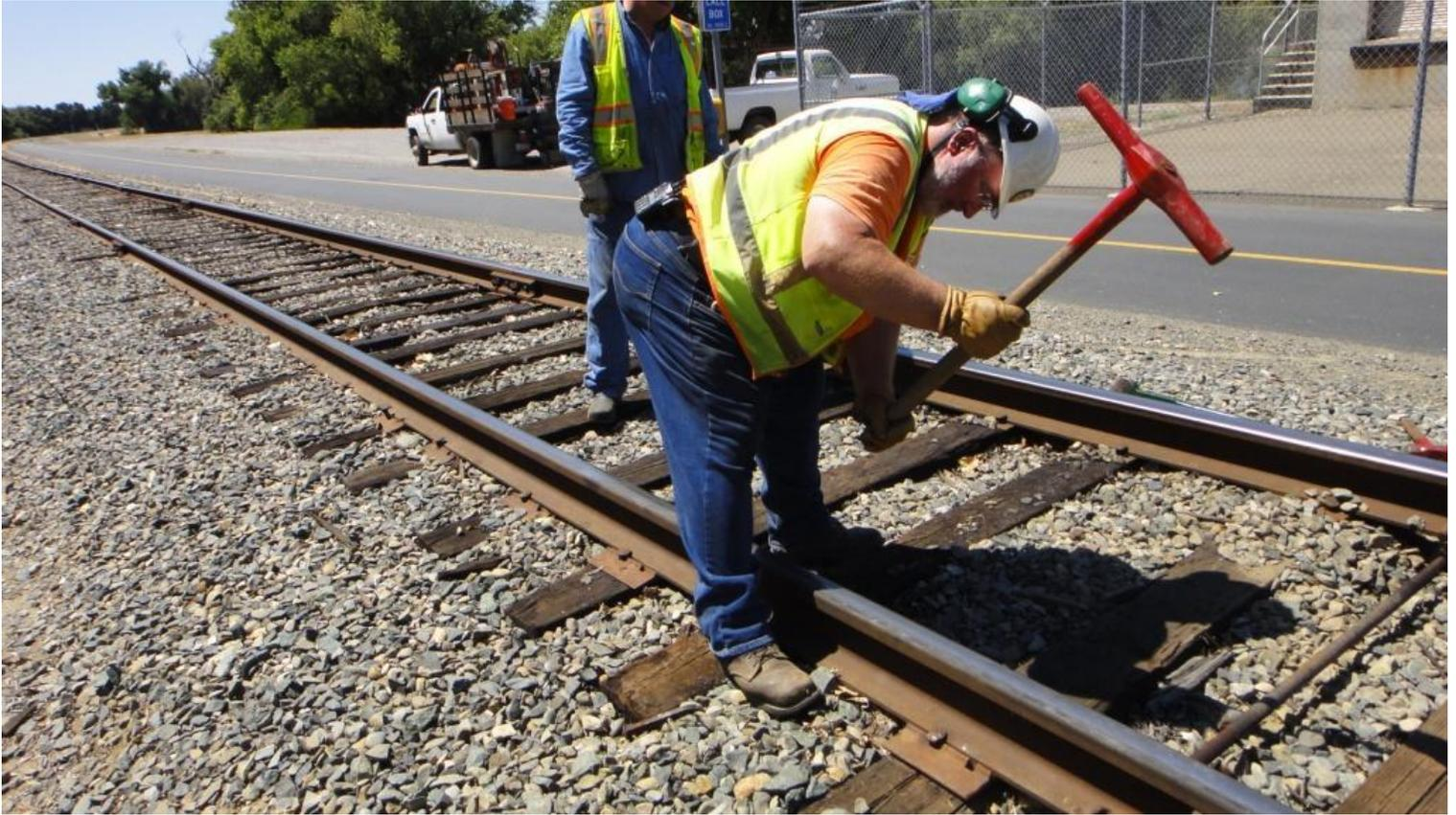
After the gauge-rods are tightened down Frank re-spikes the re-gauged track
