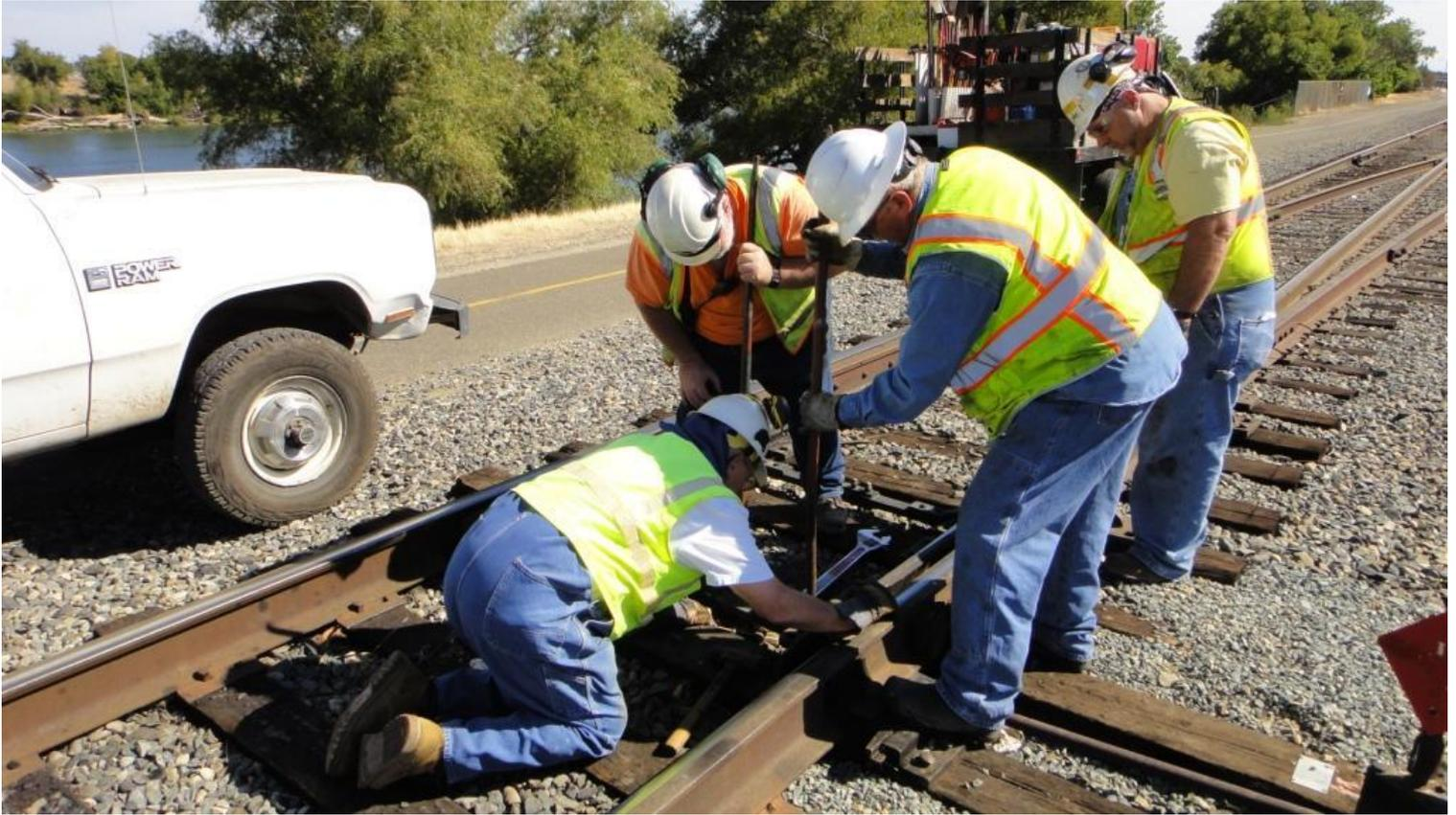
Scott uses a lining bar to adjust position of the transit clip while Frank adjusts the connecting rod. Then Clem gets the bolt in place
