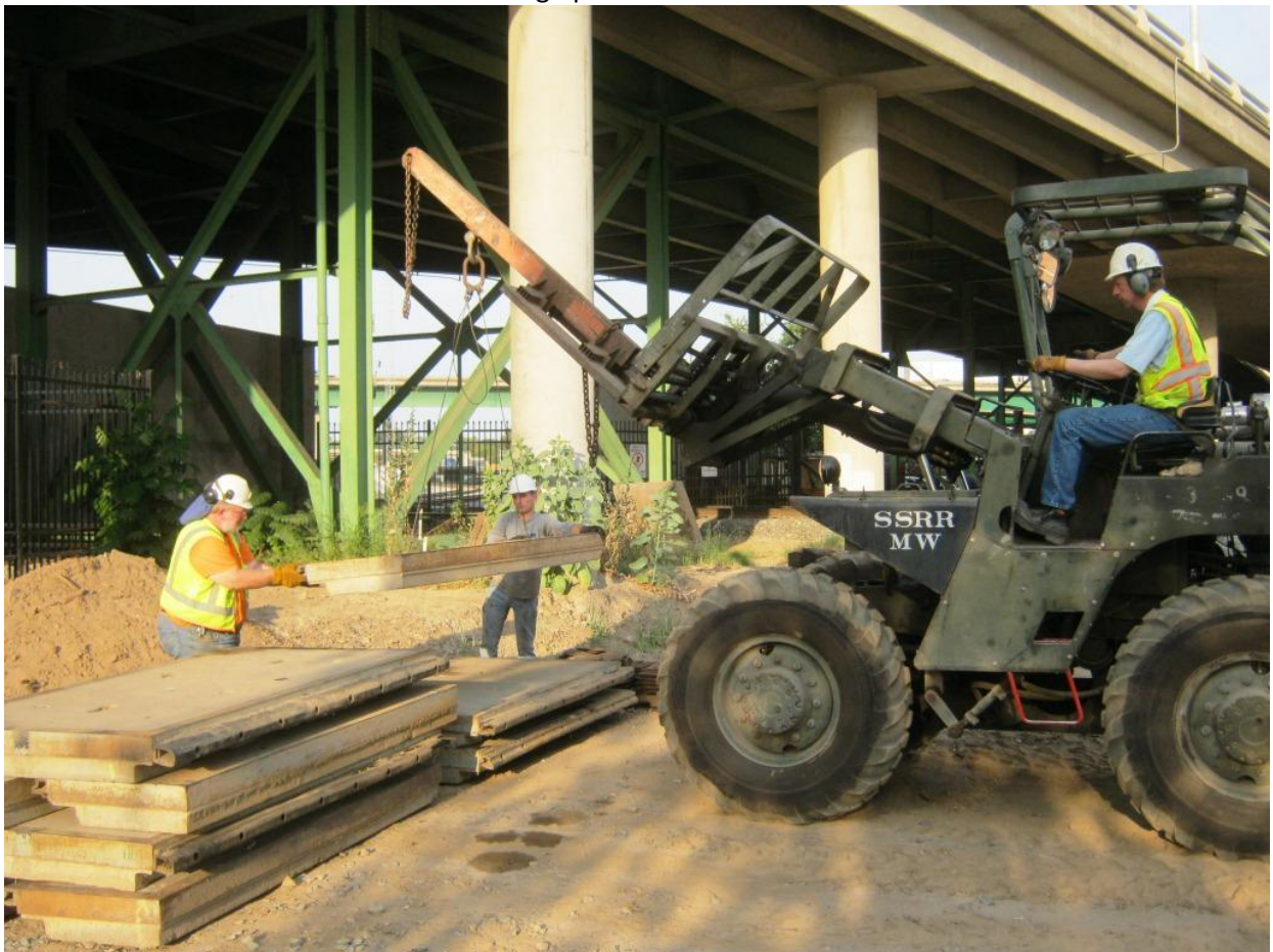
Frank and Garrick guide the concrete panels into neat piles.
