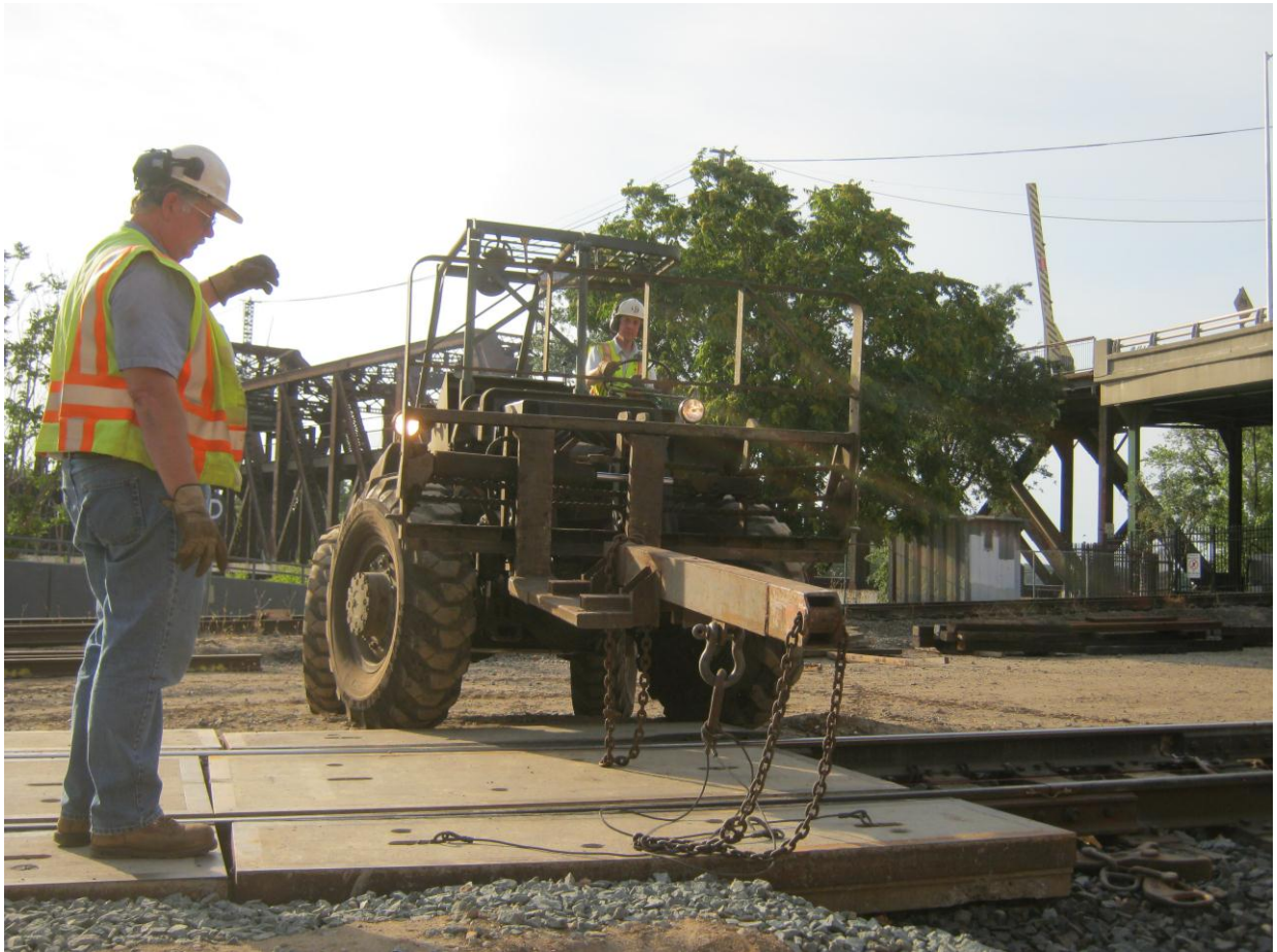
Chris directing operations on the 560 Track
