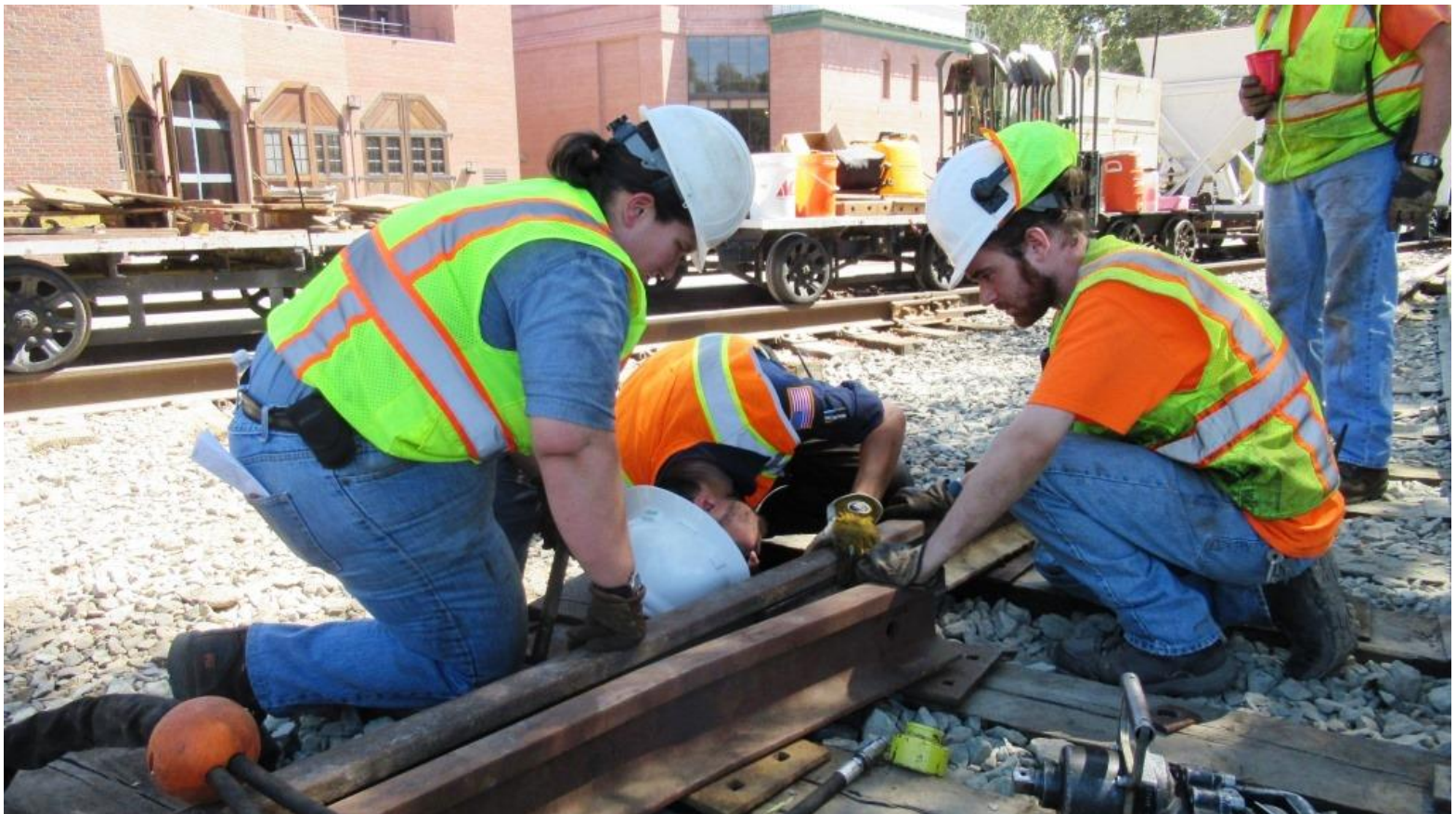
Kyle sights the bolt-holes to line everything up with Heather and Matt's help
