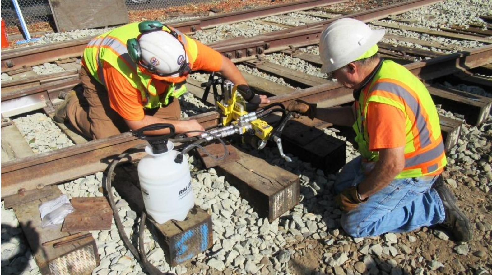
Chris and Mike H. set up the new hydraulic rail-drill which is so much easier to use than the old gas-powered drill
