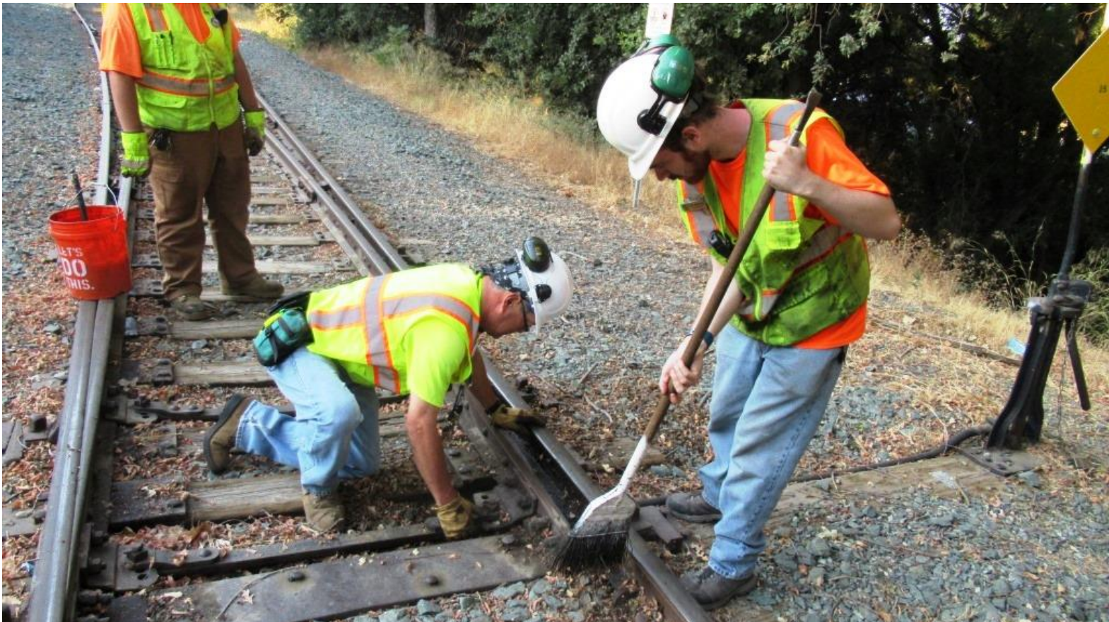
Taka and Matt clear obstructions from around the connecting rod
