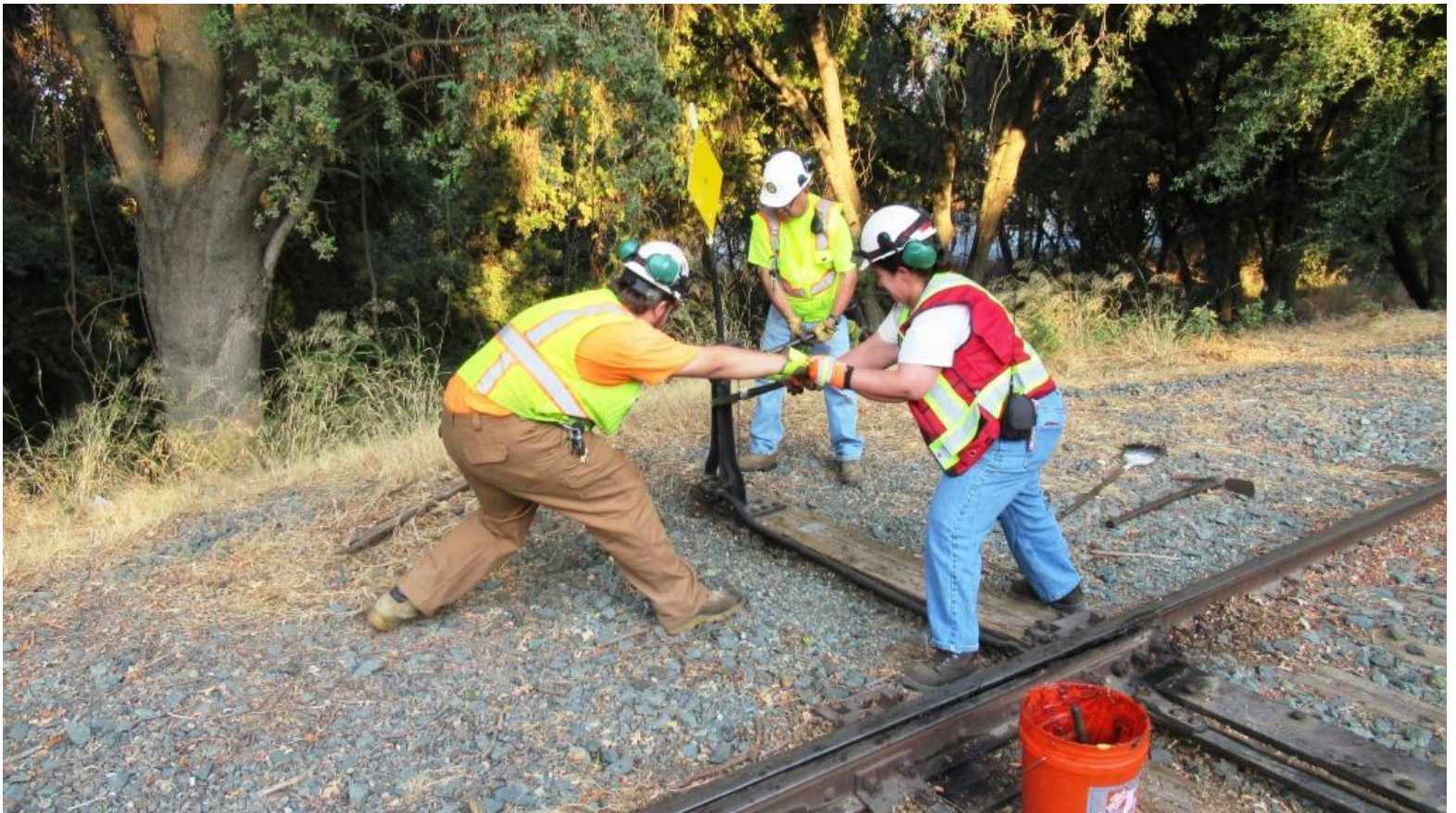
Chris and Heather use the switch-stand twisting tool to give the stand a good, old fashioned twist
