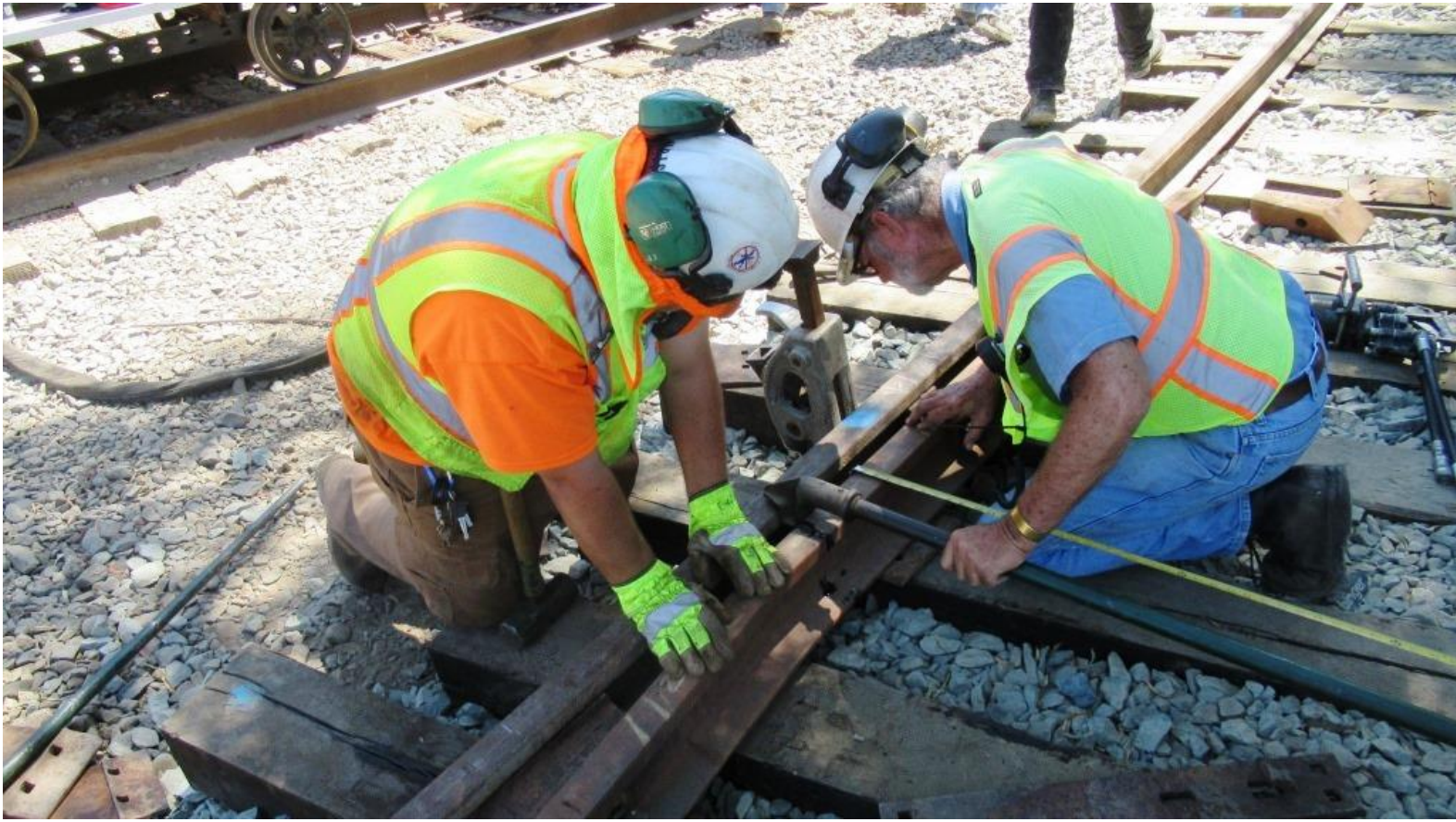
Chris and Alan checking guard-face and guard-check measurements and found that something wasn't quite right
