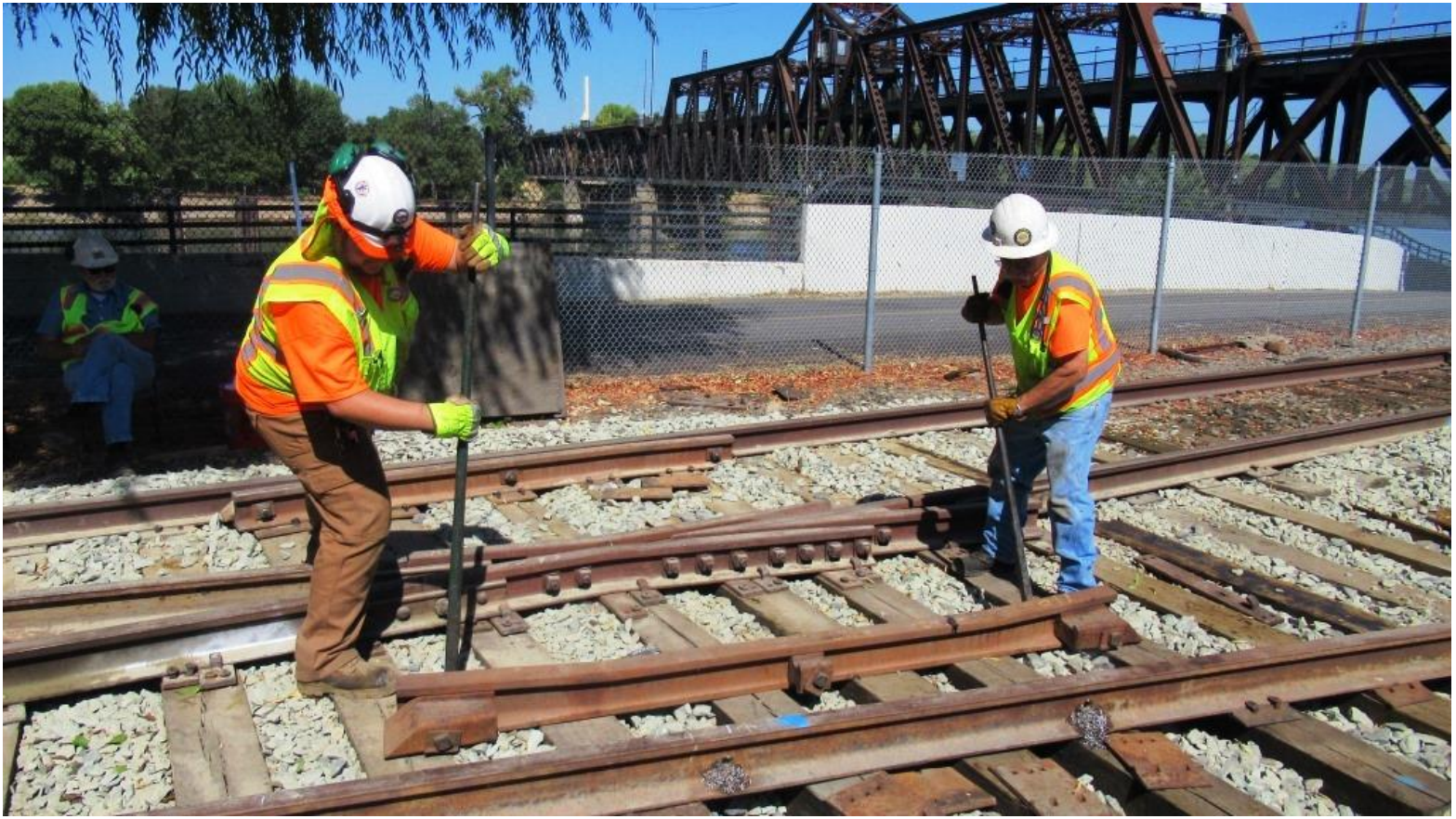
Chris and Mike H. shimmy the guard-rail into position
