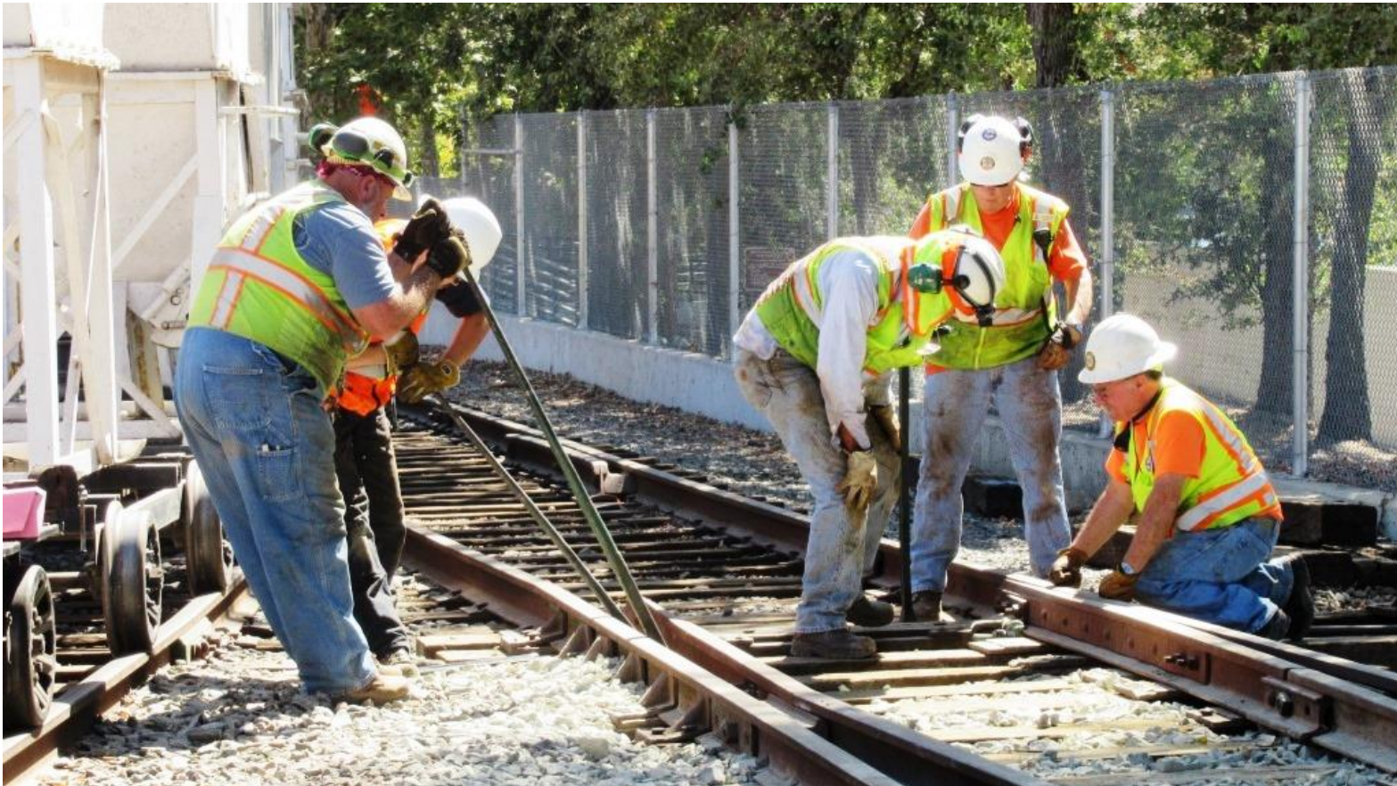
Time for the real-world test: Mike F., and Kyle lever the switch-points over to the diverging track as Steve, Bill, and Mike H. clamp it
