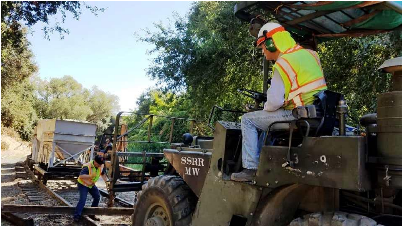
Ed M. hooks the rail-tongs to the stick of rail for Steve on Big Green to lift onto the flatcars
