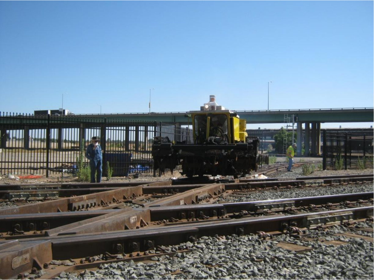
Dave Megeath piloting the Scarifer over the UP Main.
