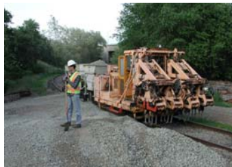
John standing on ballast in front of the ballast train.
