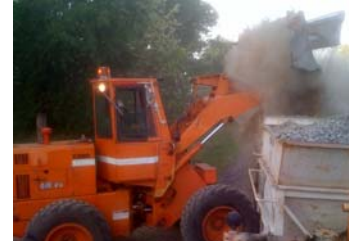
MOW Loader filling our ballast carts
