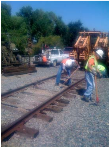
Steve and Jack working on the track.
