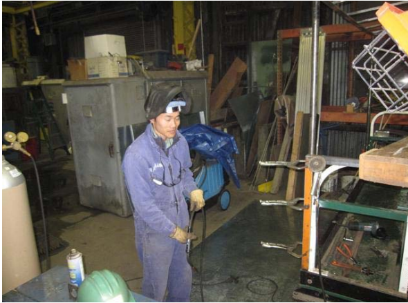
Bert is moving in to weld together more of his roof project.
