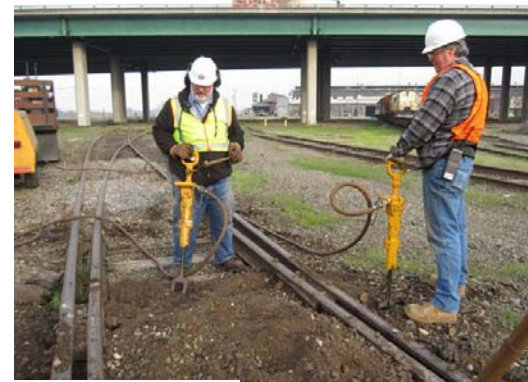
Frank and Ron on the hand tampers in the shops yard.
