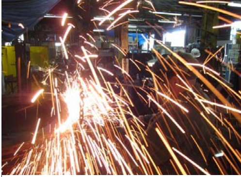
Ed, on the torch cutting off bolts.
