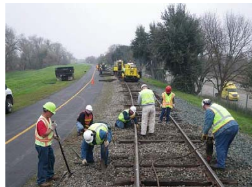
The crew plating the ties and spiking.
