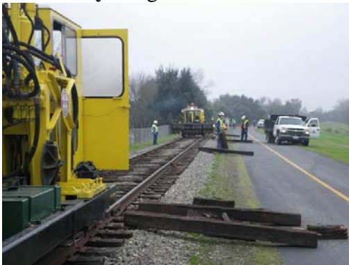
Looking back from the Shear on the Tie Gang.
