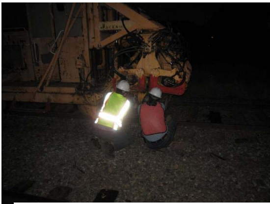
Brenton and Ron working on the tamper at Clunie.
