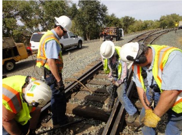
The Saturday Crew spiking one of the new 9' ties in Switch #20
