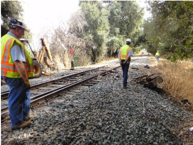
Chris and John inspecting the work on Switch # 16
