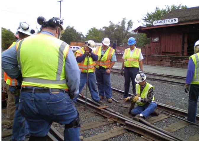
MOW crew works on the Angles Branch switch at Jamestown.
