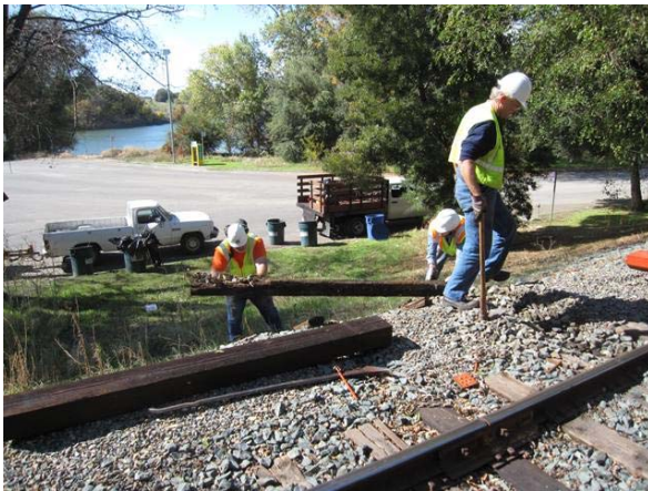
Frank, Brenton, and Steve changing ties on the SSRR mainline.
