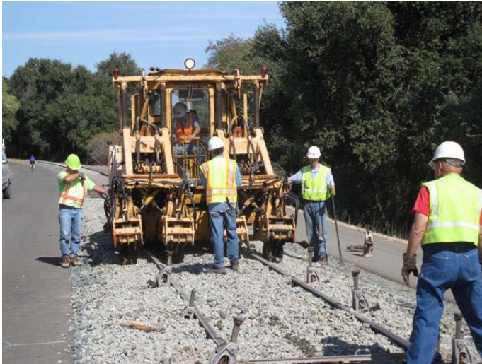
Alan Hardy at the controls of the tamper with the rest of the crew clearing jacks and directing the tamper.
