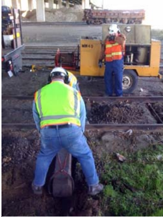
Frank inserting a new tie while Harry looks on.
