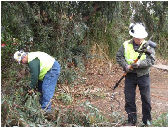
Mike and Ed trimming trees that were encroaching on the mainline.
