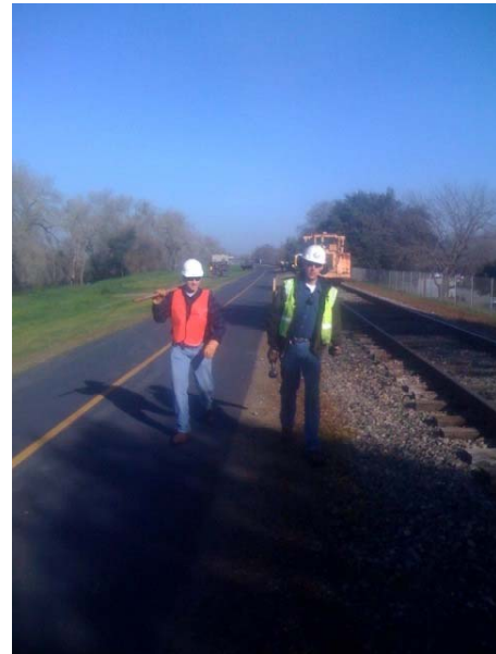
Kevin and Richard heading out to set rail anchors.
