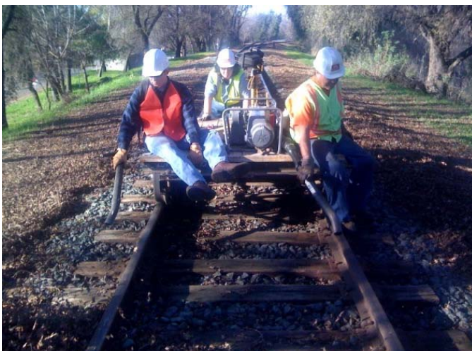
Kevin and Jon blow the leaves off the track from a motor car trailer while Heather acts as the locomotive pushing them along.
