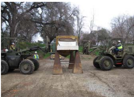
Forklifts unloading the shaker at Setzer.
