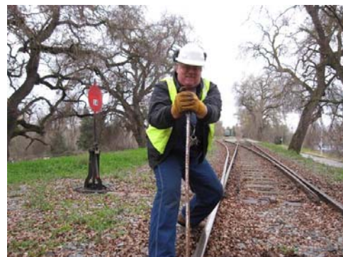
Chris tightening a bolt at Miller Park
