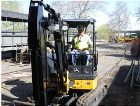
Leonard on the excavator.
