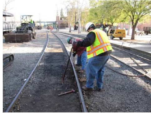
Al and Scott removing joint bars and pulling spikes.
