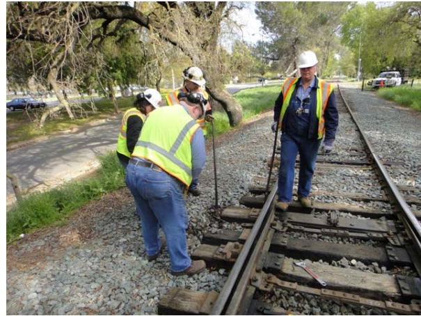
Chris, Frank, Mike and Heather work on the points of switch #14
