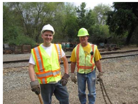
Oleg and Steve take a break for a quick photo between digging out the dumpster
