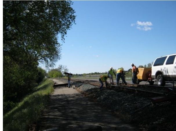
MOW crew on Saturday changing ties on the SSRR mainline at M.P. 2.2
