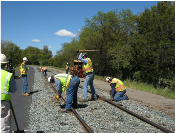
MOW crew driving spikes on new ties on the SSRR mainline at M.P. 2.2
