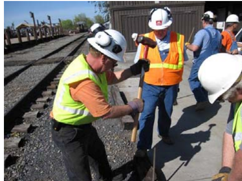
Pounding stakes to secure tie curb in Old Sac.
