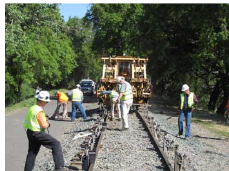
Track Raise in progress
