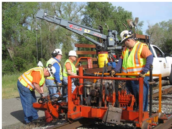
Using the Section Gang machine to change a tie at M.P. 2.8
