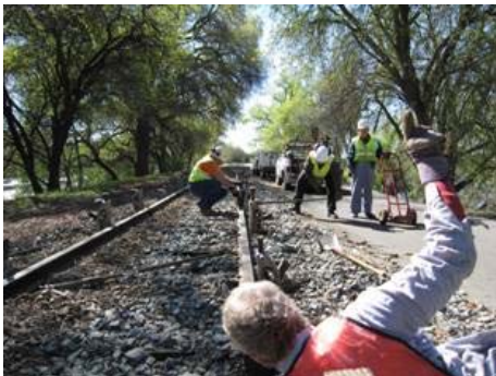
Using the spot board to raise the rail 2 inches
