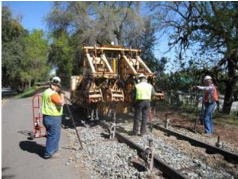
Saturday Crew Tamping the raised rail
