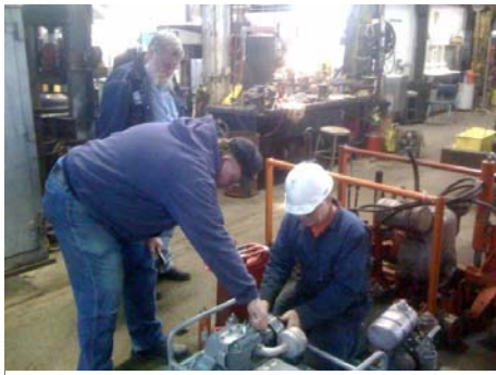
Mike and Gene working on the generators.
