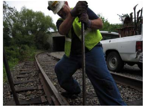
Mike tightening a bolt on Setzer spur.
