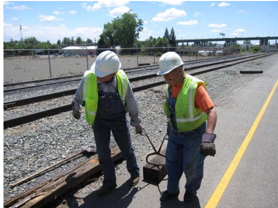
Steve and Jack moving a new tie into position.
