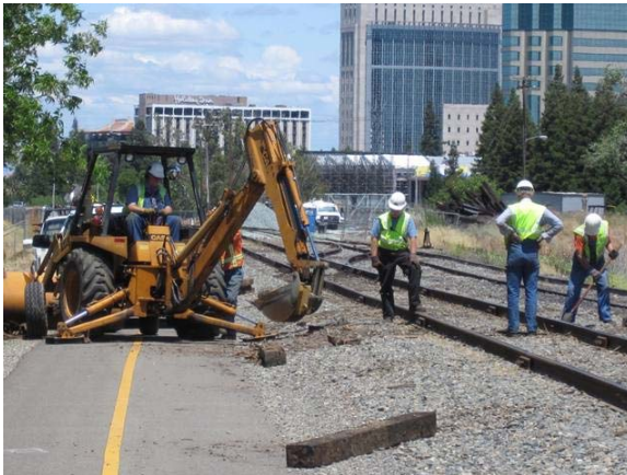
MOW Saturday crew and the backhoe working on tie replacement.
