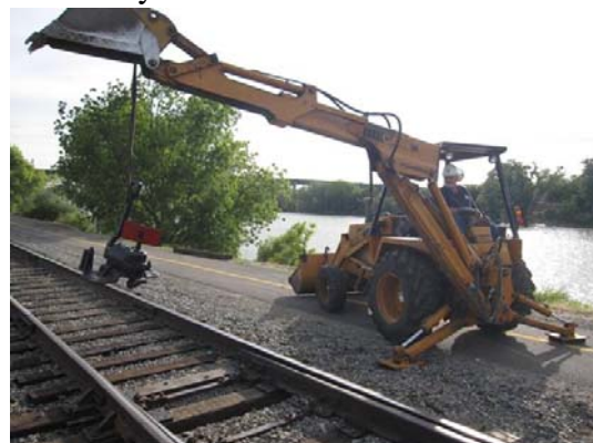
Sandy using the backhoe to position the new switch stand.
