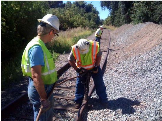
Steve holds the air hose for Mike working the spike hammer while Clem checks gauge further down the line.
