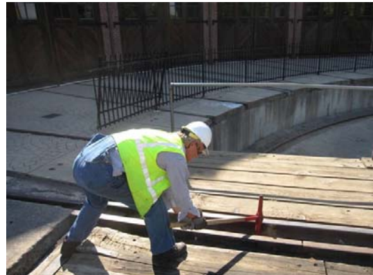
Steve driving a spike on the turntable
