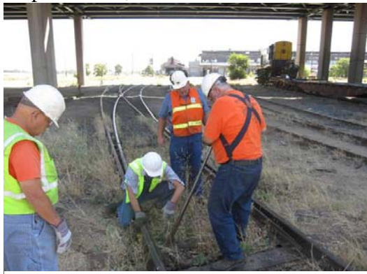
Sandy and the crew working on the yard track
