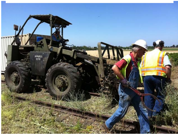
Steve N. moves into position with a tie tong ready to move ties into position in front of the container.
