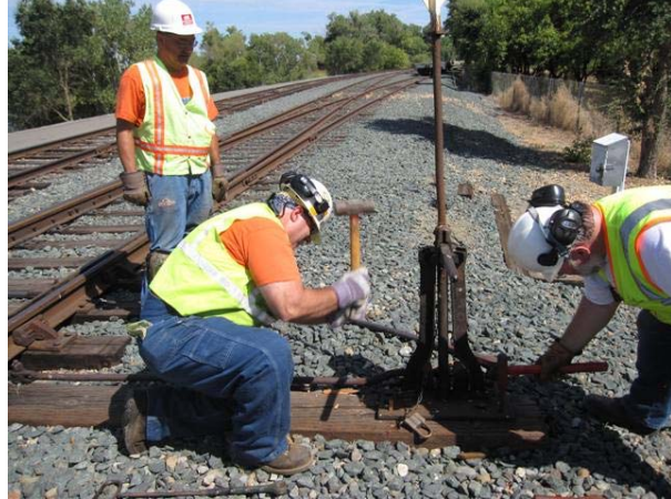
Mike is setting a spike in the switch stand while Frank inserts tie plugs. Jon stands watch ensuring they guys do a good job.
