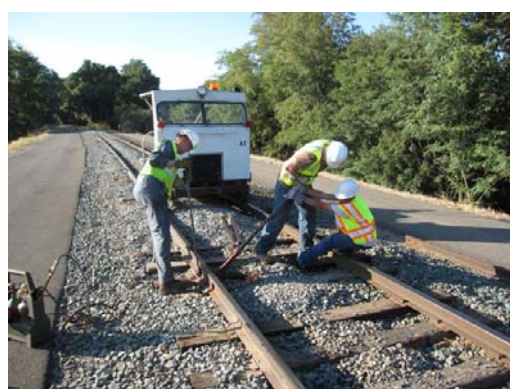
Richard, Caleb, and Brenton working to remove the old rail.
