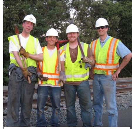
Tuesday rail change out crew.
