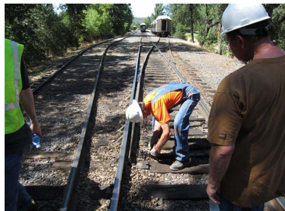
Steve working on a switch at Railtown
