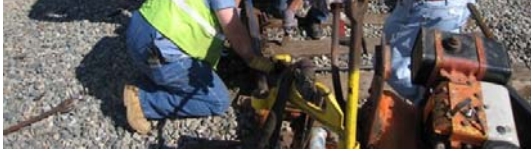
Crew pulling off joint bars for greasing.
