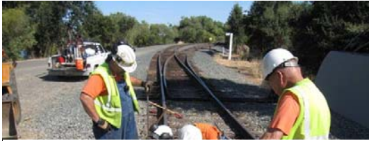
Crew pulling off joint bars for greasing.
