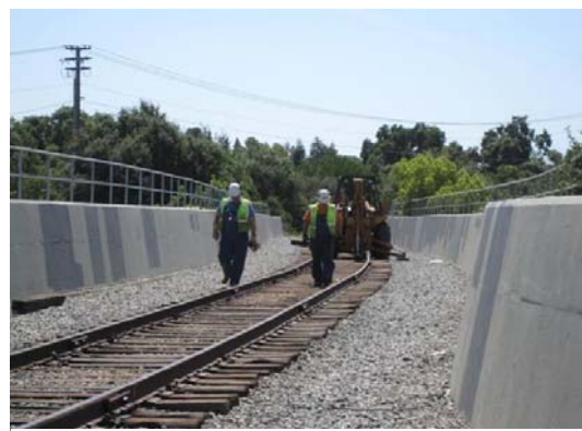
Chris and Mike inspecting the bridge track.
