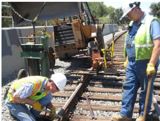
John and Chris use the torch on a tough track bolt.
