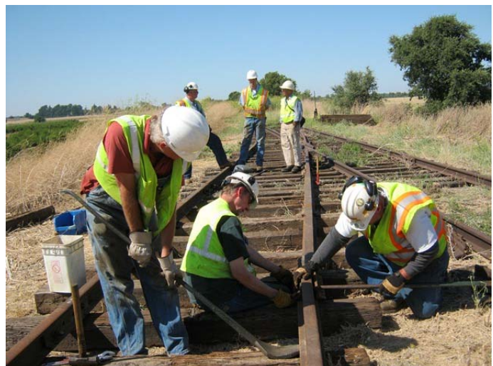
Steve and Mike line up the joint bar holes so Richard and place the bolt. In the background, Chris, John, and Mike discuss butterflies or something.
