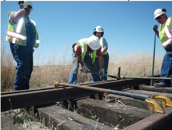
Chris and Harry supervise while Heather nips the tie for Steve as he drives a spike. Yes that is a track gauge so we are doing this property.
