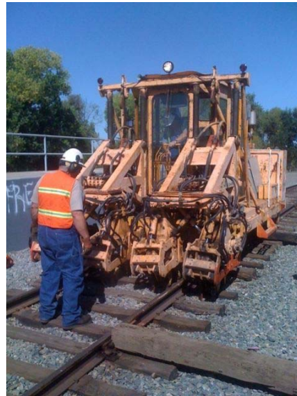
Harry directs Chris Carlson in the Tamper as he tamps the track.
