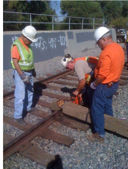
Harry cuts a tie to use for jacking with the help of Chris Talbert while Jack supervises the work.
