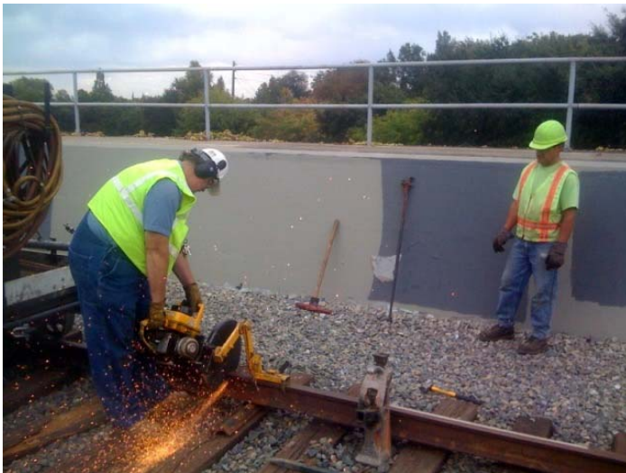
Chris trimming the rail to fit while Steve supervises the work.
