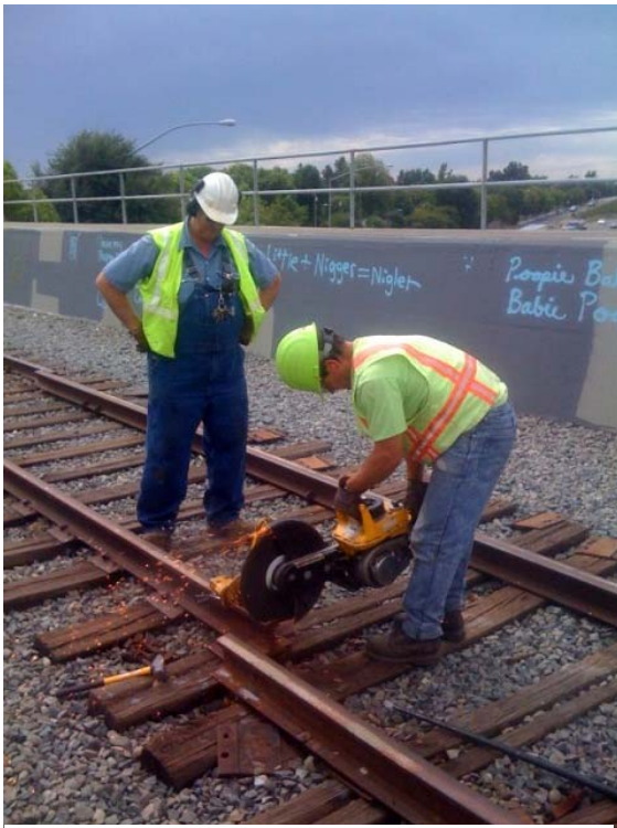
Steve trimming the other end of the rail while Chris supervises.
