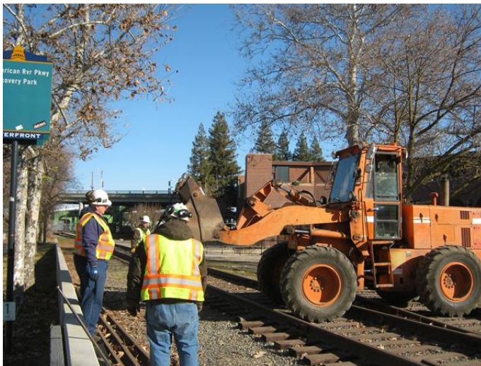
Harry, Richard, and Mike guide the loader in to remove rail from Old Sacramento that had been resting along the tracks for years.
